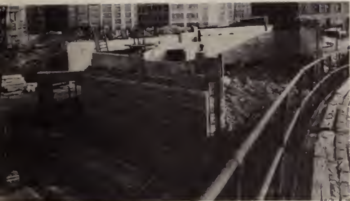
View shows the east wall of Prospect Street under construction, as it appeared in December, 1952.
